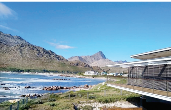
It features a Grapa wooden deck and ceilings, a saltwater pool, and frameless sliding doors, allowing for “seamless indoor-outdoor living”
